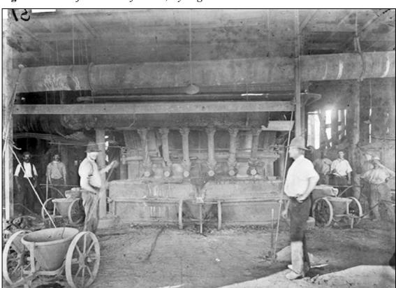
Figure 3: Water jacket blast furnace, Nymagee mine ca. 1900.
