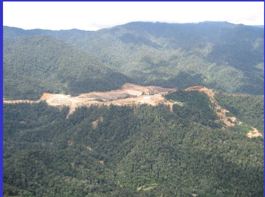
Tailing Dam construction
