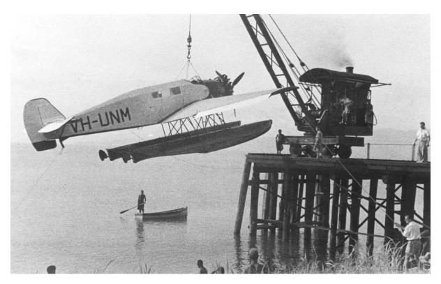
The crane at Lae was pivotal to Bulolo Gold Dredging's success. It ran on railway tracks linking the jetty at Voco Point to the aerodrome a distance of 1,200 yards. The water at Lae was too deep for the construction of a jetty capable of mooring large ships, so ships had to stand offshore, loading everything onto lighters. The crane would then unload the lighters before conveying everything to the aerodrome where it would in due course load them onto aeroplanes for Bulolo and Bulwa.
